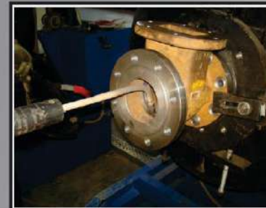
MECHANIZED SEAT RING SEAL WELDING SYSTEM
